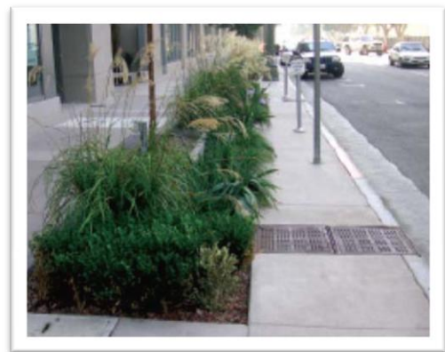
Parkway Infiltration Swale 11th St & Hope St – Los Angeles
