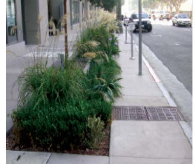
Parkway Infiltration Swale at 11 th St & Hope St – Los Angeles
