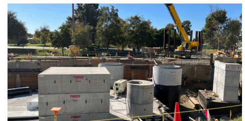
Adventure Park Multi Benefit Stormwater Capture Project: stormwater capture project with an underground cistern, funded by the Safe, Clean Water Program. The project is shown here under construction (far left and far right), and ensuring proper tree protection (center). Photos by: Heal the Bay.
