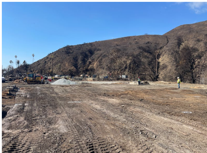
Photo of the Palisades staging area under construction.
