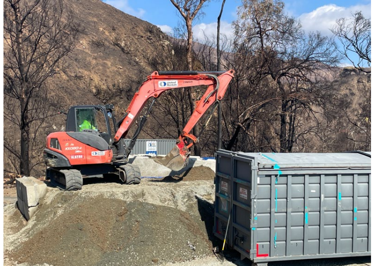
Photo of the Palisades staging area under construction.
